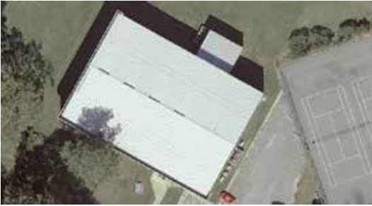
Figure 3b. The natural color image showing a metal roof building (as seen in Figure 3a) at NASA Langley Research Center. **
